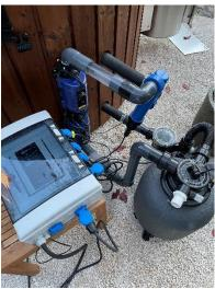
Since April, the photovoltaic power manager AC•THOR from my-PV has been heating the jacuzzi with solar electricity.
