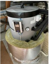
Another AC•THOR controls the heating of the 200-liter tank for the house's hot water supply.
