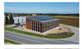
Building's reversed concept: The solar modules predetermined the design of the outer facade.
